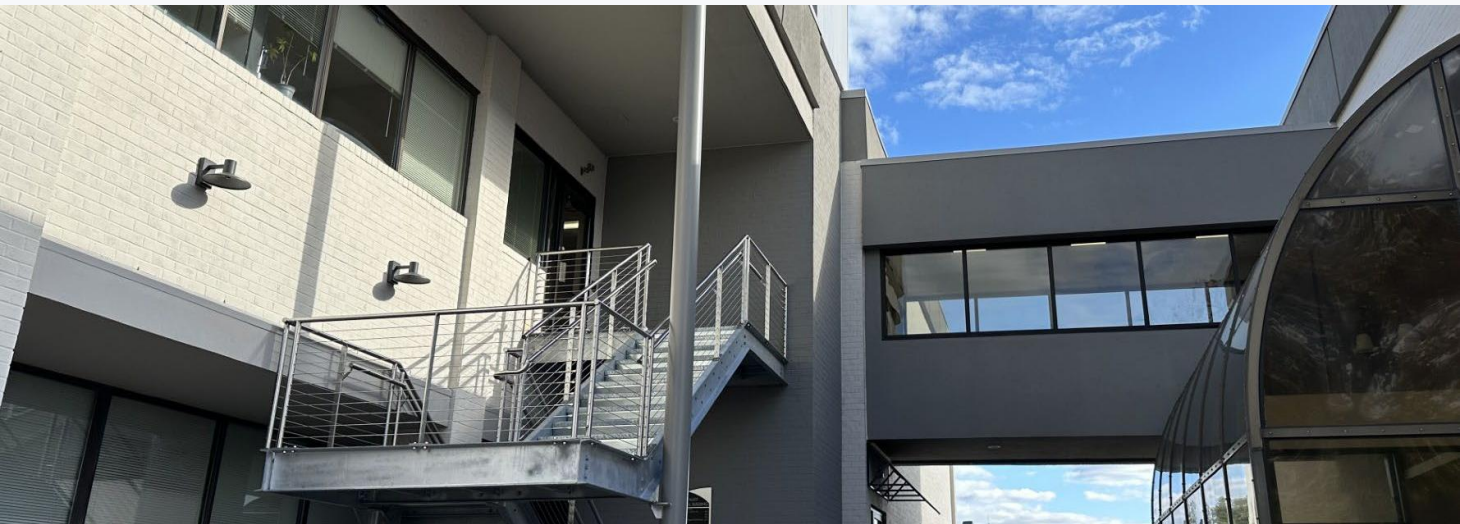
COURTYARD & COVERED WALKWAY
